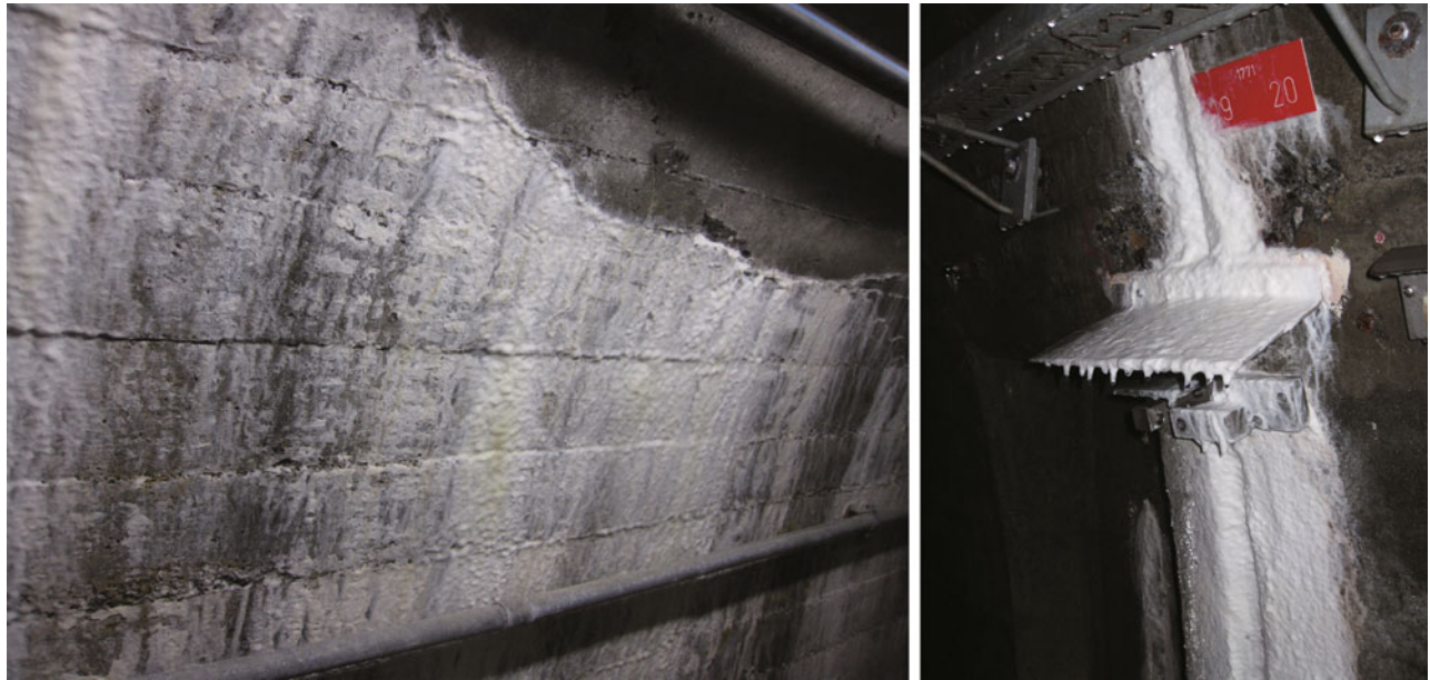
Fig. 10 Efflorescences in control galleries at crack (left) and at joint meter location (right)
